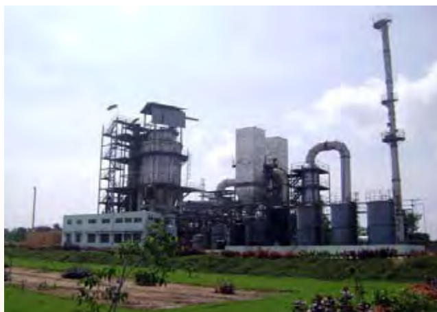
FIGURE 11: HAZARDOUS WASTE INCINERATOR
